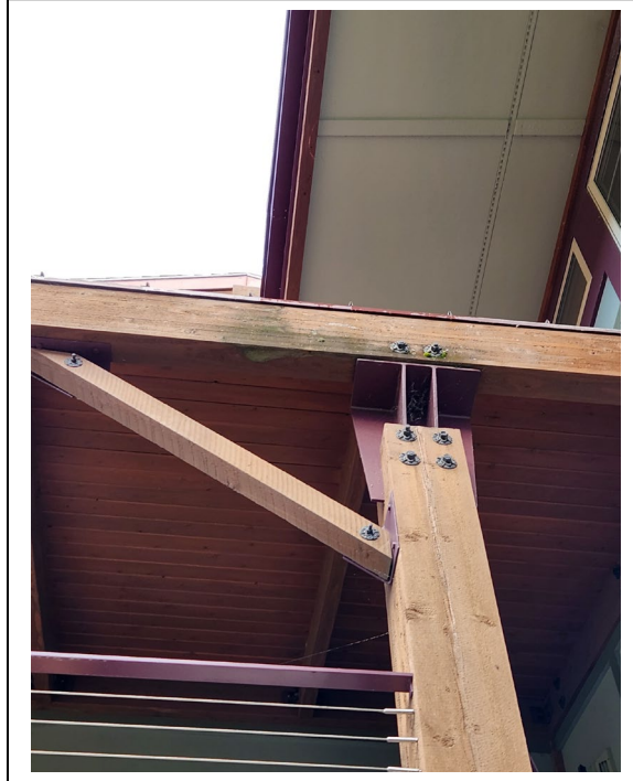
Figure 2-8: Unit 202 Roof Edge
